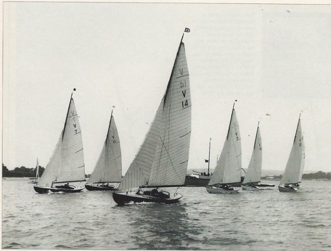
Left: Pictured soon after the start of a race in 1934, the Solent Sunbeams, each with distinctive house racing flag, focus on the first mark. Note the high, looping tiller and narrow panelled sails of the era. The boom of the nearest yacht is sheeted almost over the centreline and she is making good ground to windward with her tall rig.
